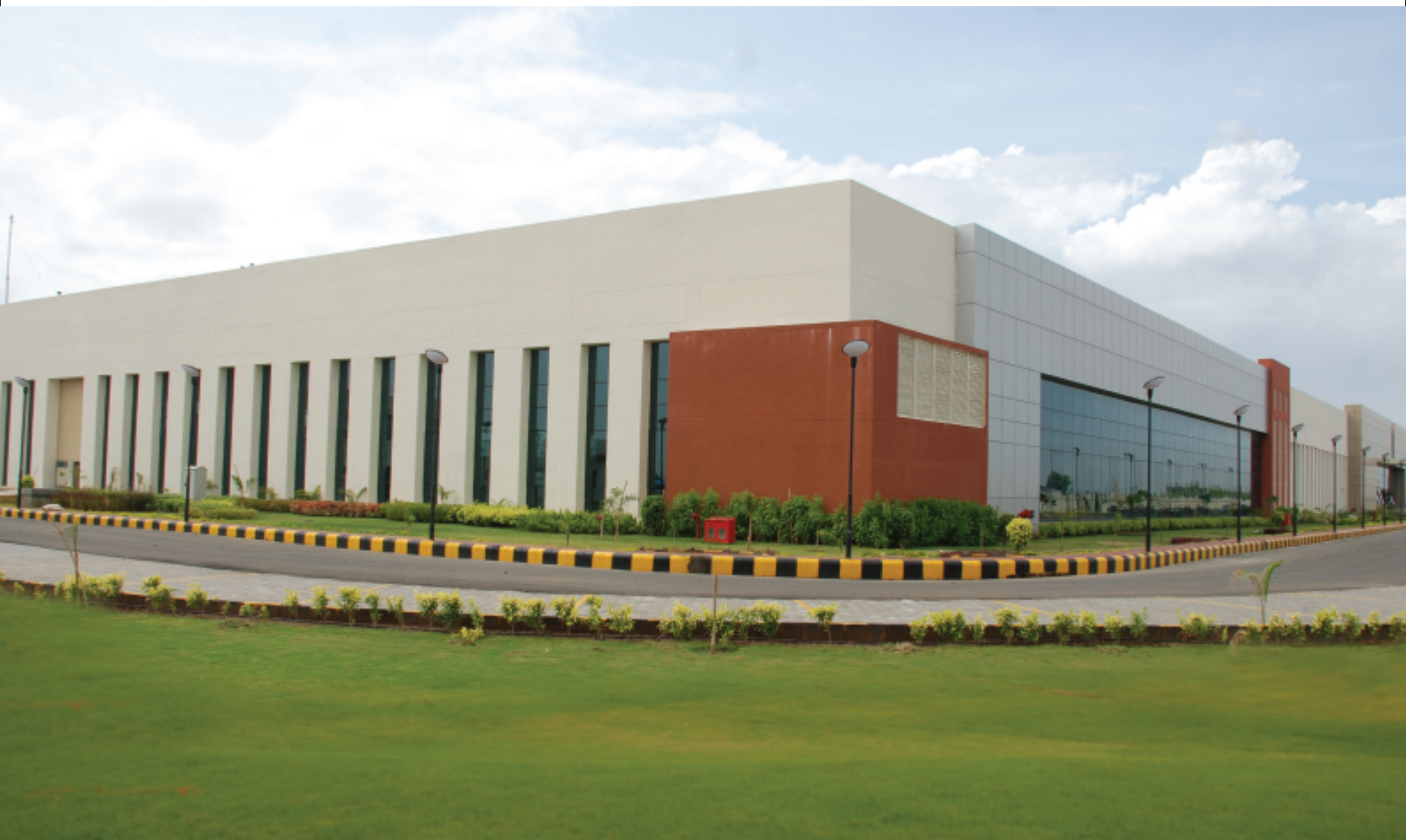
Switchgear Factory, Baroda
