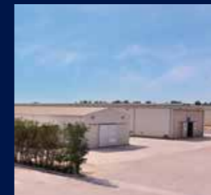
Jubail, Saudi Arabia Integrated Manufacturing Facility
