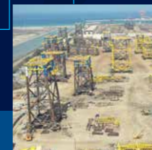
Sohar, Oman Modular Fabrication Yard
