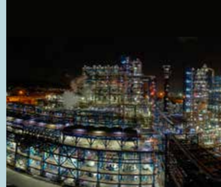
Crude Distillation and Vacuum Distillation Unit (CDU & VDU) Capacity: 9 MMTPA | EIL
