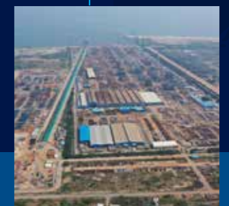
Kattupalli, India Modular Fabrication Facility
