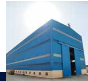
Jubail, Saudi Arabia Heavy Wall Pressure Vessel Facility
