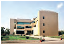
Administrative Building, LTSSHF, Hazira
