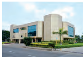
SBU Block (2nd floor), Hazira
