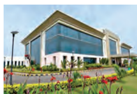
Administrative Building, Vadodara
